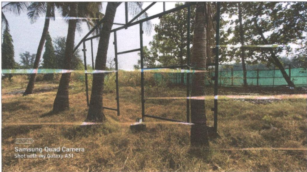
Pic 11: Metal frame existing at the site.
